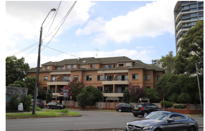
Figure 9 North west elevation of 2 Wilson Street fronting the site (Photographs - Urbis)
