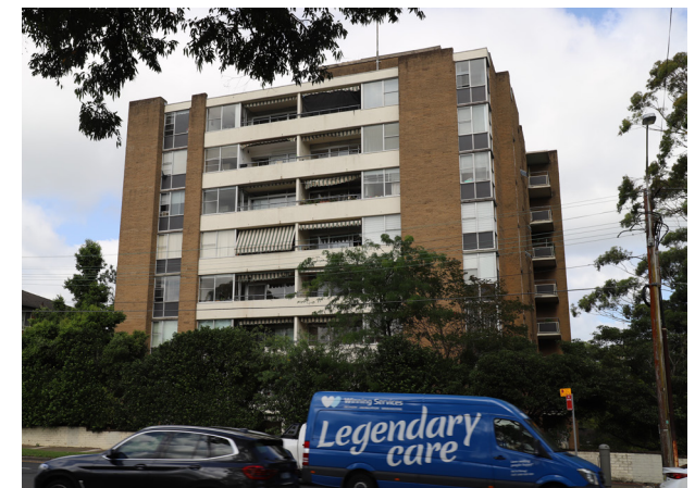
Figure 17 East elevation of 856 Pacific Highway (Photograph - Urbis)
