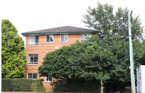
Figure 16 East elevation of 854 Pacific Highway
