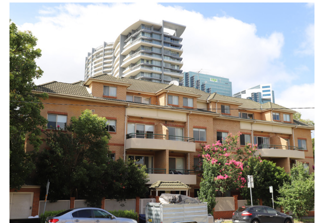
Figure 10 North Elevation of 2 Wilson Street (Photographs - Urbis)
