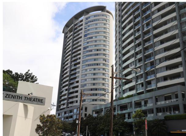
Figure 13 South and west elevation of 11 Railway Street and part elevation of 9 Railway Street (Photograph - Urbis)
