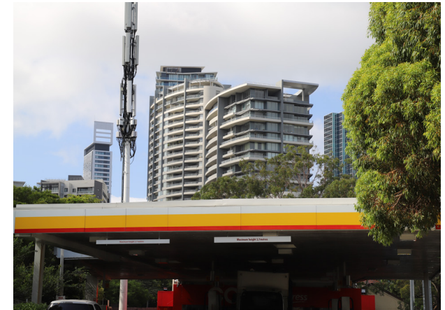
Figure 12 North elevation of 11 Railway Street from Pacific Highway (Photograph - Urbis)
